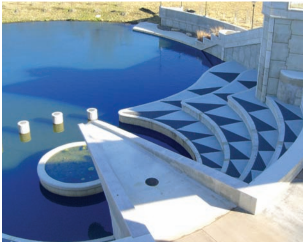
LAKE LENEXA DAM AND SPILLWAY Lenexa, Kansas
