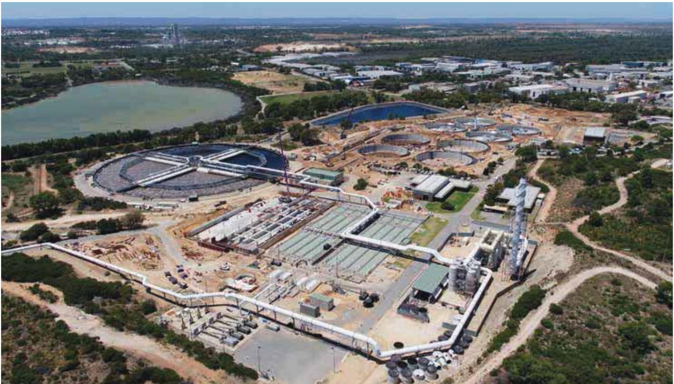
Effective planning enables the Water Corporation in Western Australia to develop and maintain sustainable water supplies. Upgrades to the Woodman Point Wastewater Treatment Plant in the Perth metro area will increase treatment capacity and the quality of treated wastewater, which is used to produce recycled water for industry use. Photo by WP180 Alliance
